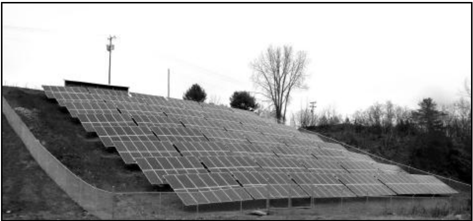
Cavendish Municipal Solar Array shown here in late November during construction
